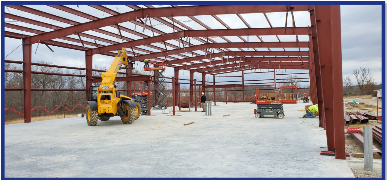
New ECC Support Building Under Construction
