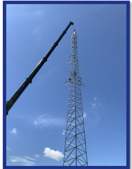
New Tower Site Construction
