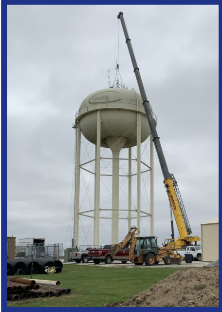
Redtail Site Antenna Work
